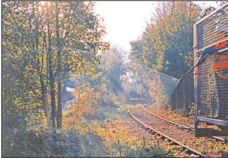
(Above) The operator riding in the trailer can spray selectively using a hand-held lance. (Below) Similar procedure is possible using the Land Rover unit. (Bottom right) Fixed off-track spraying can cover a five-metre swathe.
